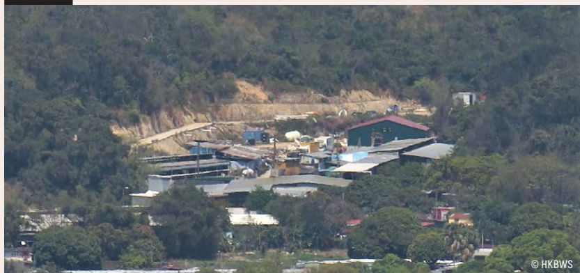
The cut slope and site formation work at Tai Kong Po which was suspected to have intruded into Lam Tsuen Country Park and is related to a STT granted by the LandsD
