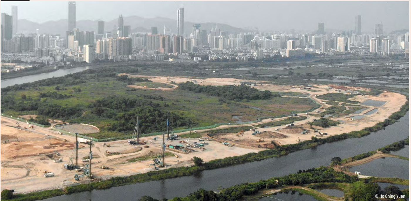
Some of the advance works at Lok Ma Chau Loop encroached into the wetlands and fenced off areas
