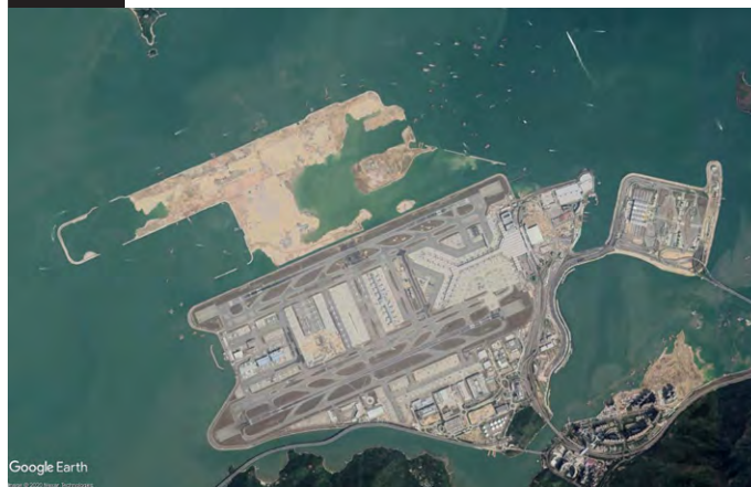
Google Earth aerial photograph taken on 17 February 2020, showing the reclamation works and the associated marine traffic for the airport’s third runway and the Tung Chung East extension.
