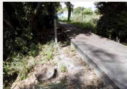
(Credit: John Allcock / WWF-Hong Kong) – Caption “Drop in soil level along the AFCD path.”
