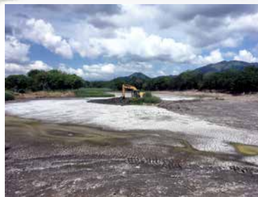
Restoring the island (Credit: WWF-HK)
